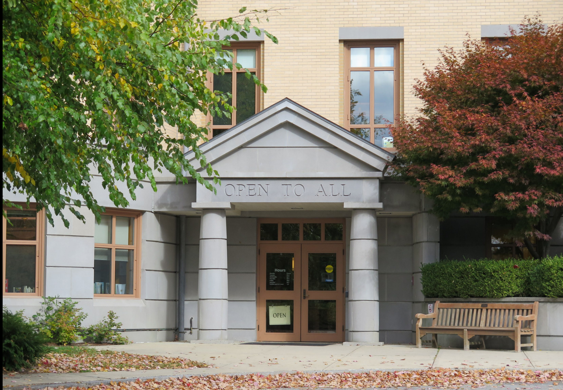
New accessible entrance – now truly “Open to All” 1999
