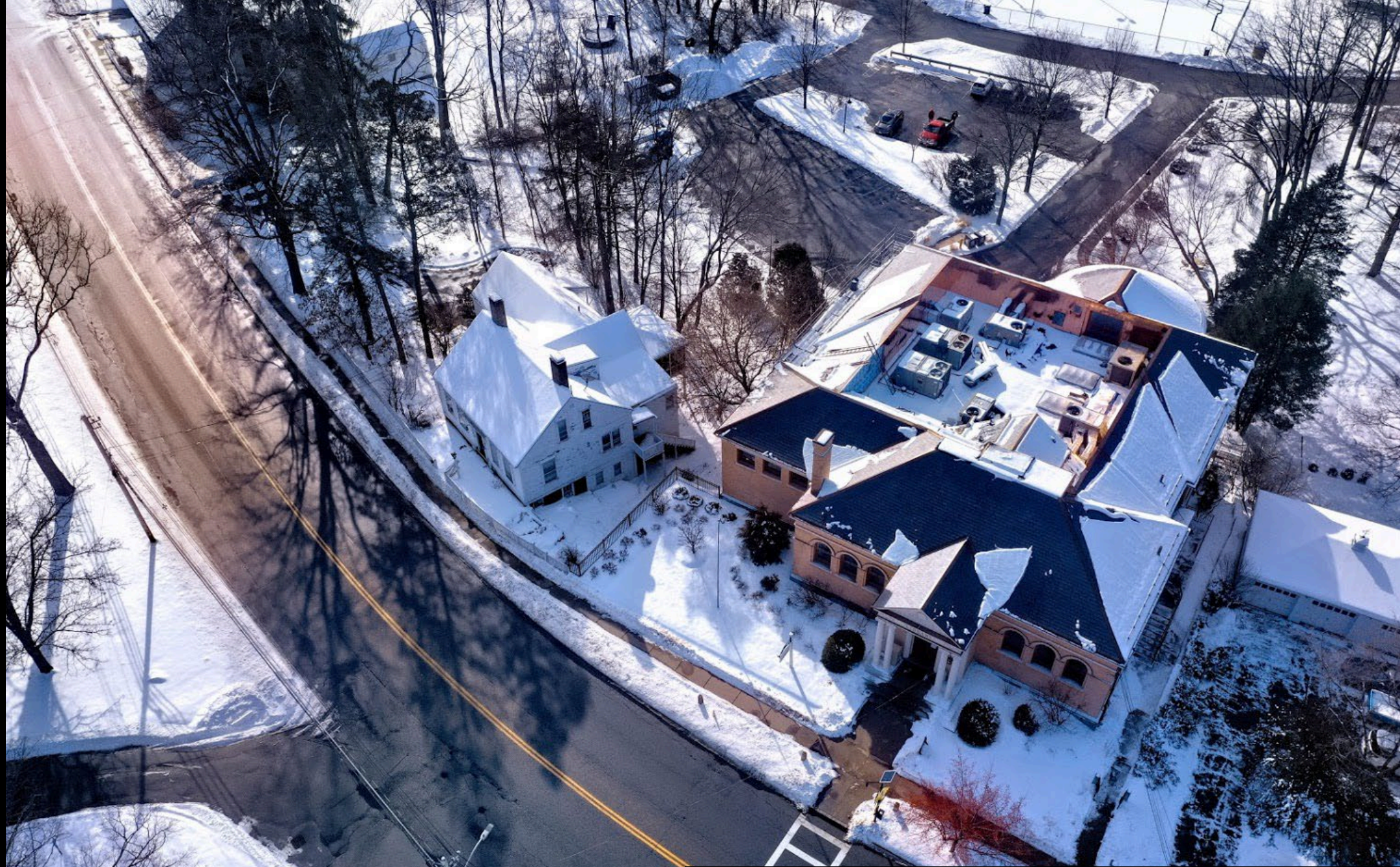
4,000 to 17,000 sq. ft.! Aerial view of our beloved library 2020
